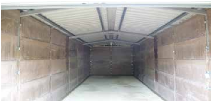
Fibre Cement Roof Finishes
