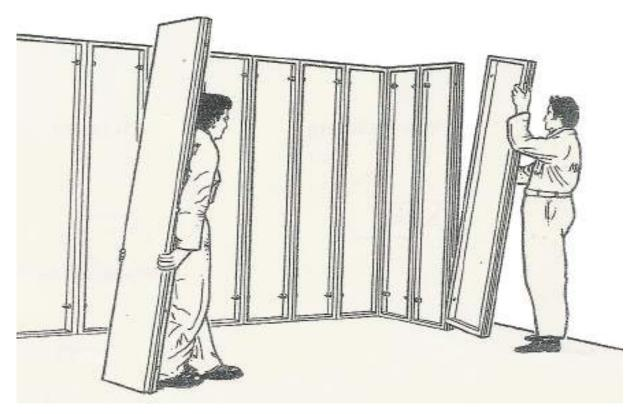
Starting in the **LEFT** hand **REAR CORNER** assemble your corner using the **HEEL AND TOE** method of assembling, assemble 3 panels either way loosely, then using a **SPIRIT LEVEL** upright your panel and tighten the bolts ensuring that the tops are flush against each other.
